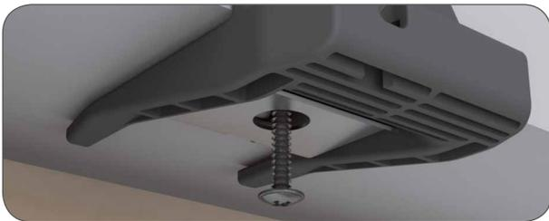
3. Keeping the tool in place, either drill a pilot hole through the centre of the holes on the bracket, or - if fitting to a suitable substrate - directly drive a screw up into the recess until tight. Ensure the tool stays flat and square against the recess while doing this. Once the screw is tight, the tool can be pulled out of the bracket.
